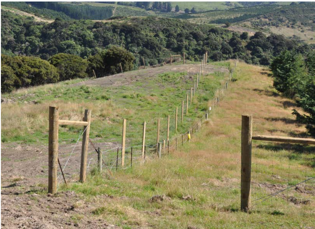
Figure 2. Deer fence being installed along the Tiromoana Bush boundary.
