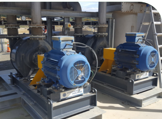
These blue pumps are like a vacuum cleaner that sucks the gas out
