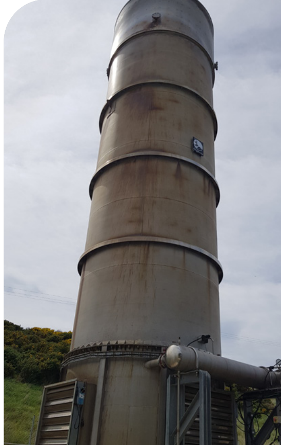
The chimney that burns off excess gas
