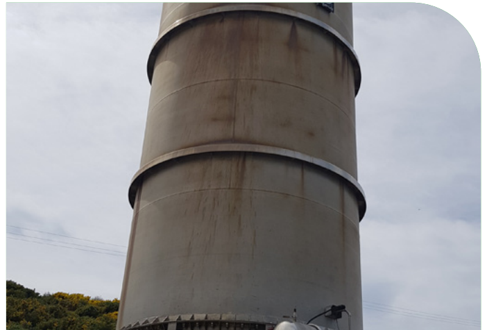
Any gas that can't be turned into electricity is burnt off in this flare
