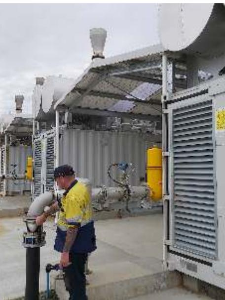
The gas extracted from the Landfill is mainly methane (50-60%) and carbon dioxide. Transwaste is committed to capture and destroy methane in line with New Zealand's Emissions Trading Scheme. While burning the gases would destroy them, there's a better option and that's to use methane as a fuel to run internal combustion engines and produce renewable energy - electricity - the option Transwaste chose.
