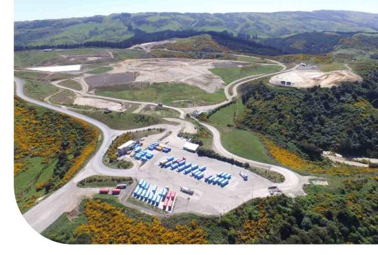
The design and operation of the Kate Valley Landfill addresses all the known environmental risks and concerns. In addition to being built on impermeable siltstone, the Landfill has a multi-layered liner that completely seals the base and sides of the Landfill.
