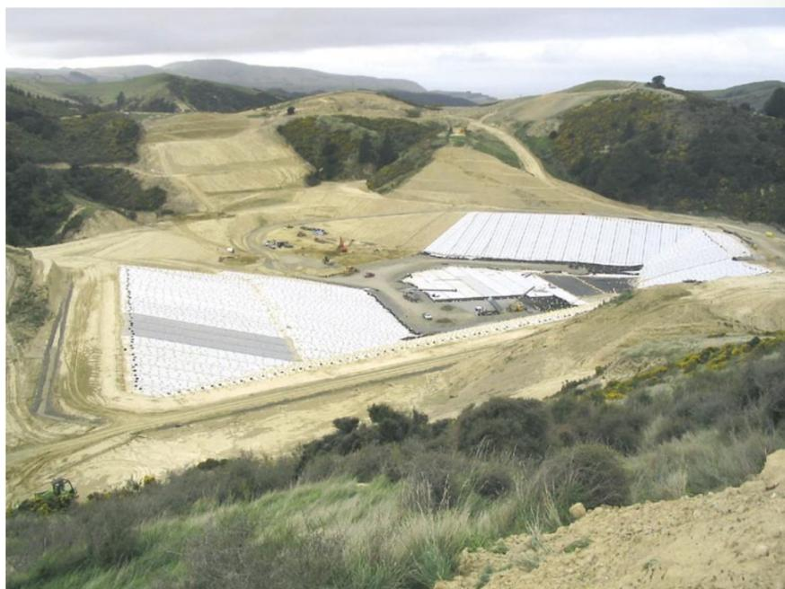
Gravel protection layer being laid on top of liner
