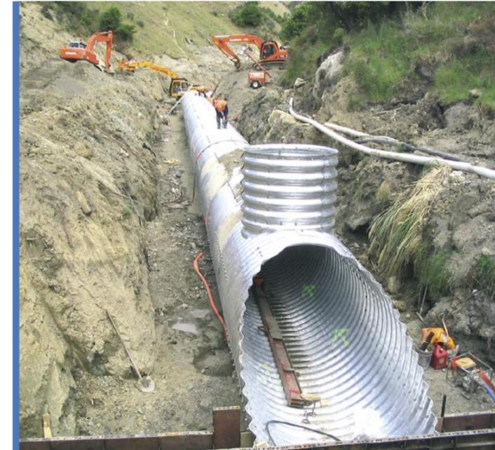
New culvert on Landfill Access Road under construction
